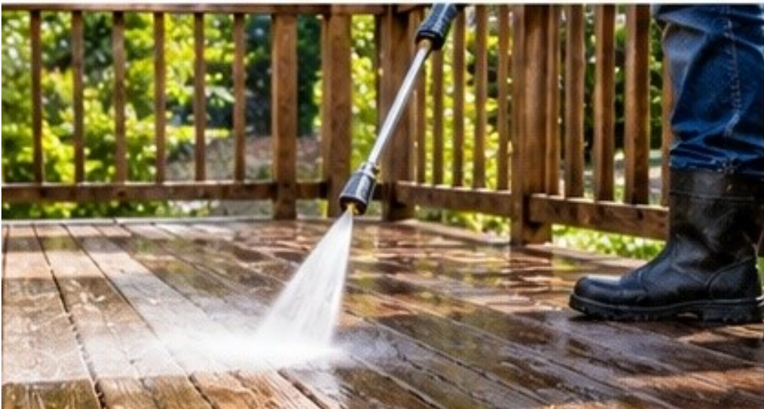
Wood and composite surfaces can be damaged by excessive pressure; test methods and follow product guidance.
