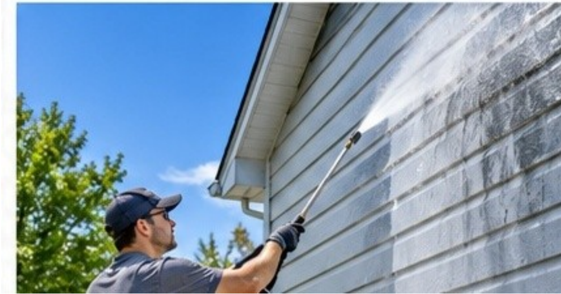
Different surfaces require different pressure, chemistry, dwell time, distance, and rinse technique.
